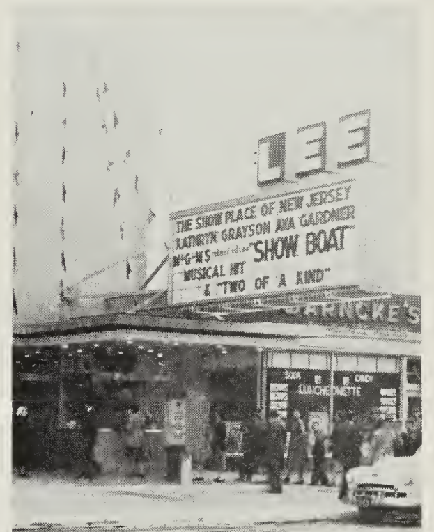
In keeping with the uncluttered design of the Lee, the stainless steel marquee, above, is of plain but attractive lines. California stucco covers the front. At left are the display frames, having perforated masonite inner backgrounds.
